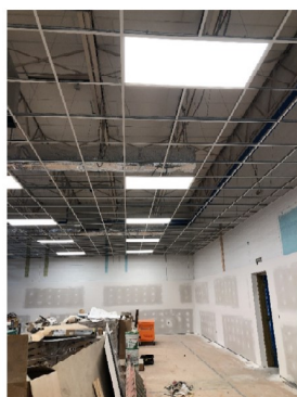
Ceiling Grid Installation at Chestnut Hill
