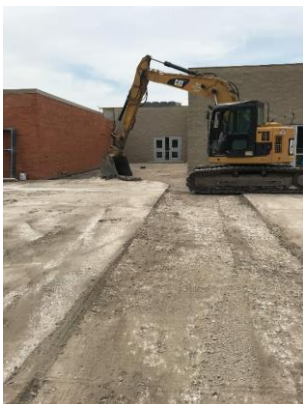
Slab excavation at Woodcrest
