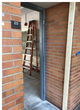
Door frame installation at Siebert
