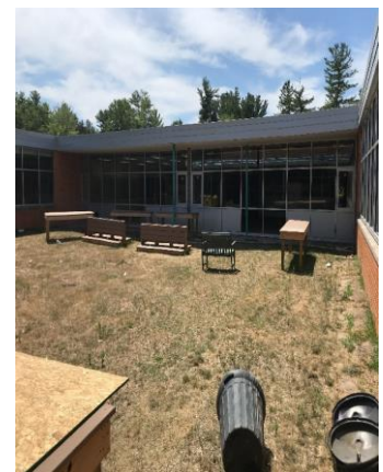
Aluminum framing and glazing installed at Siebert Courtyard
