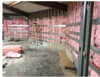
Insulation being installed at Siebert Art Room
