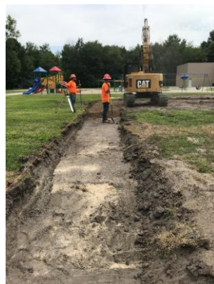
Curb preparation at Woodcrest
