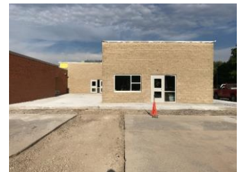
Concrete placed at Woodcrest
