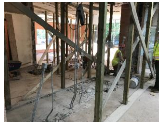
Siebert Main Office demolished
