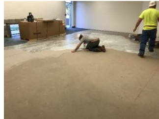
Siebert carpet floor preparation
