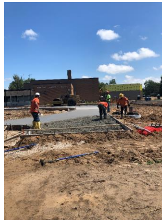
Sidewalk concrete placement at Chestnut Hill
