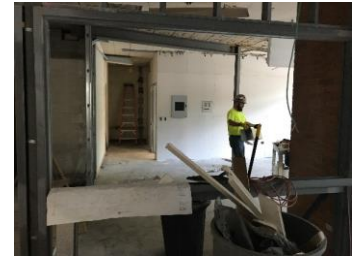
Drywall installed at Siebert Main Office
