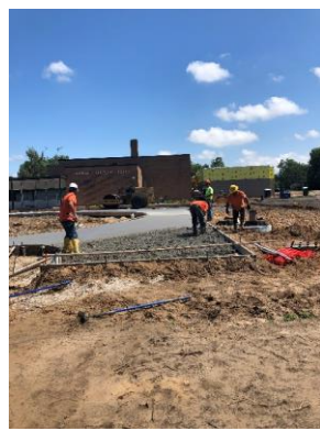
Sidewalk concrete placement at Chestnut Hill
