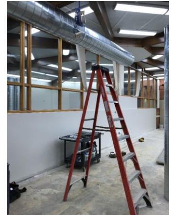
Ductwork installation at Siebert Maker Space
